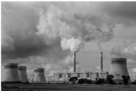
Coal-burning power station
